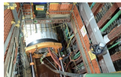
Trenchless construction achieving one of the world's longest tunnels
