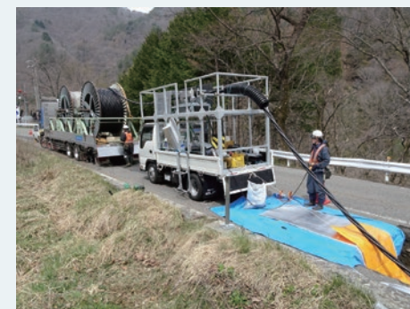
Underground cable laying and connection work
