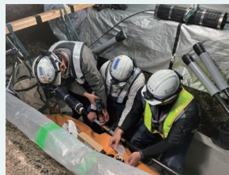
Extra-high-voltage cable connection work
