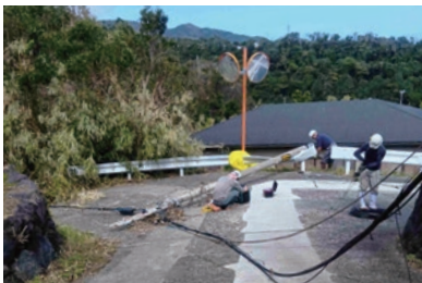
Utility pole restoration work
